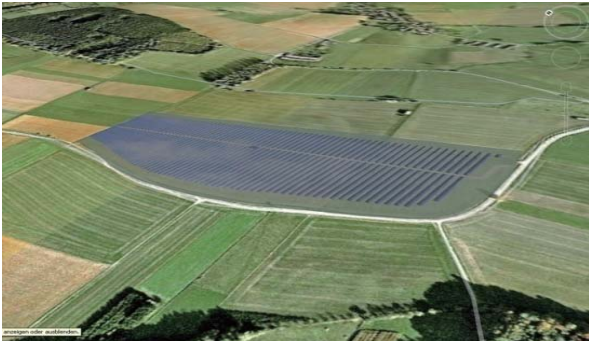
Ground Mounted 4MWp installation
